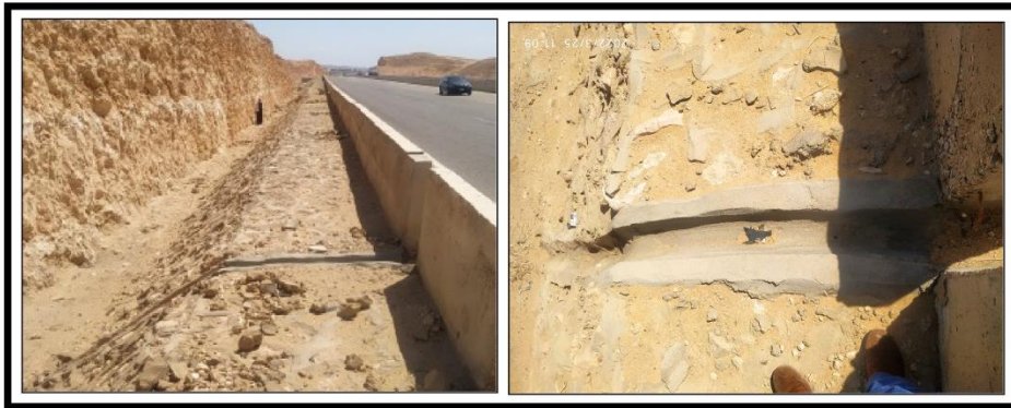
Fig. 25: Methods of Protection against the Hazards of Flash Floods on the Roads of Wadi Abu Daraj
