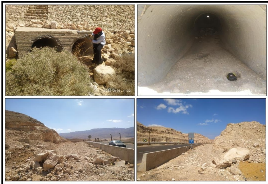
Fig. 30: Lack of Purification and Maintenance of Protection Methods against Flash Floods from Sediments and Vegetation on the Sides of Roads in Wadi Abu Daraj
