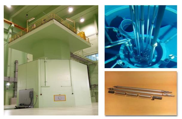
Fig. (1): Experimental Hall and reactor bloc (left) / TRIGA fuel elements and Reactor core (right)
