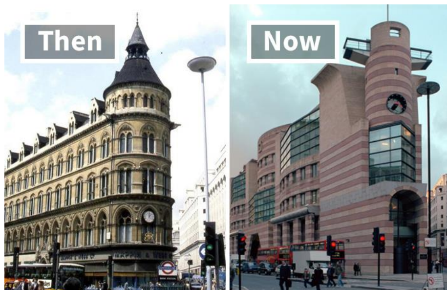
Figures 1 and 2 show a building that had been unsuitably redesigned
