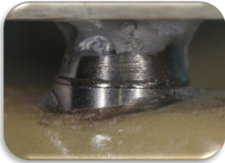
(Figure 11): Verification of proper metal-to-metal contact.
