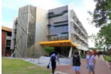
Figure (1): Australian Engineering Pavilion (Building 216)
