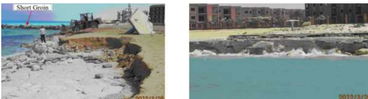
Figure 8: The loss of beach replenishment sand. Figure 9: The beach became very steep forming a scarp
