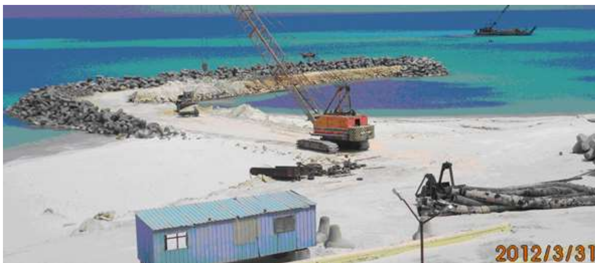
Figure 11: The artificial lagoon for executing utilities.
