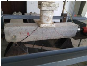
Figure 9: Failure of (CC)
