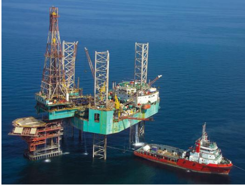
Figure 3: The jack-up platform and its supply vessel.
