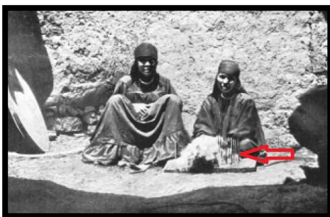
(Fig. 6) Hackling the flax through a comb with metal teeth. Location: Nahya, Giza. © (Crowfoot 1931: PL. 21).
