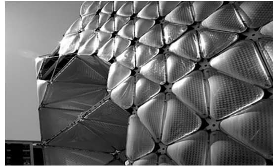
(Figure5) Smart envelope comprised of ETFE encased solar-activated lamella shades developed for the Media-TIC building in Barcelona, Cloud 9 Architects, (Hadeer Samir, 2010)
