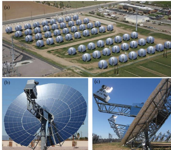
Fig. 1 (a) Overview of the Maricopa DSCSPP, Peoria, Arizona, USA (J. Coventry et al); (b) Commercial unit-scale Sun Catcher DSPS for the Maricopa DSCSPP (V. Visa et al); (c) View of the PCU for the unit-scale Sun Catcher DSCSPPS.
