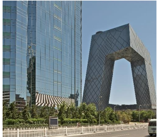
Fig. 10 CCTV Headquarters in Beijing. [15]
