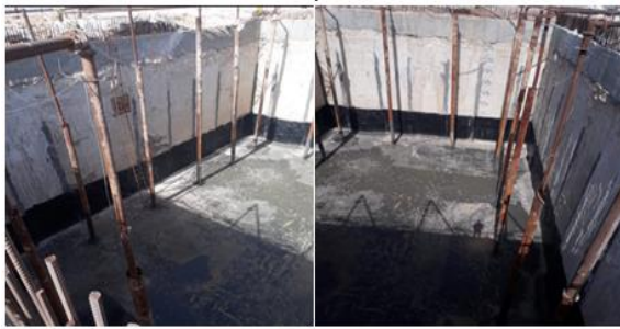
Fig 13: the diaphragm wall shaft after construction of plastic secant pile.
