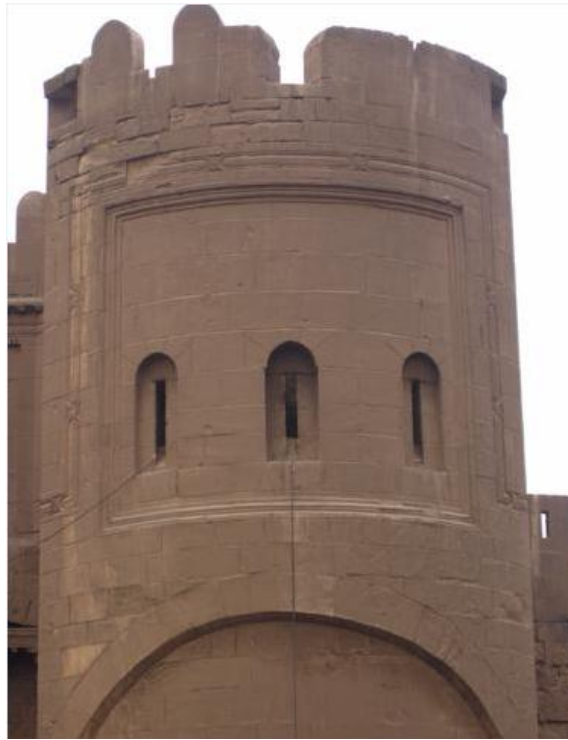
(Plate 3- Machicolations of Bab Al-Futuh Tower - Photographed by the Researcher)
