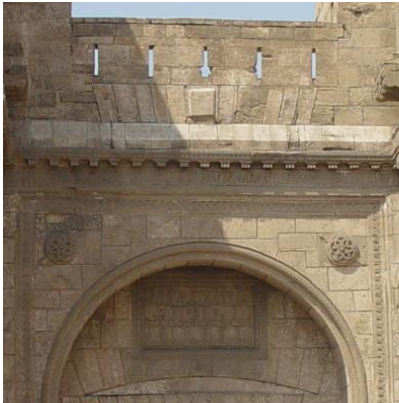
(Plate 9 - Five Machicolations to throw arrows surmounting the semi-circular arch above the entrance to Bab al-Nasr - Photographed by the researcher)
