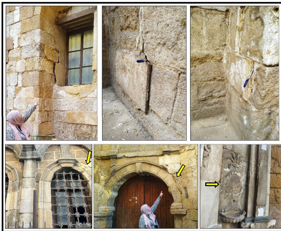
Figure 19: The Detachment and Falling of Stone Blocks, Decorations and Ornaments in Sabil Muhammad Ali
