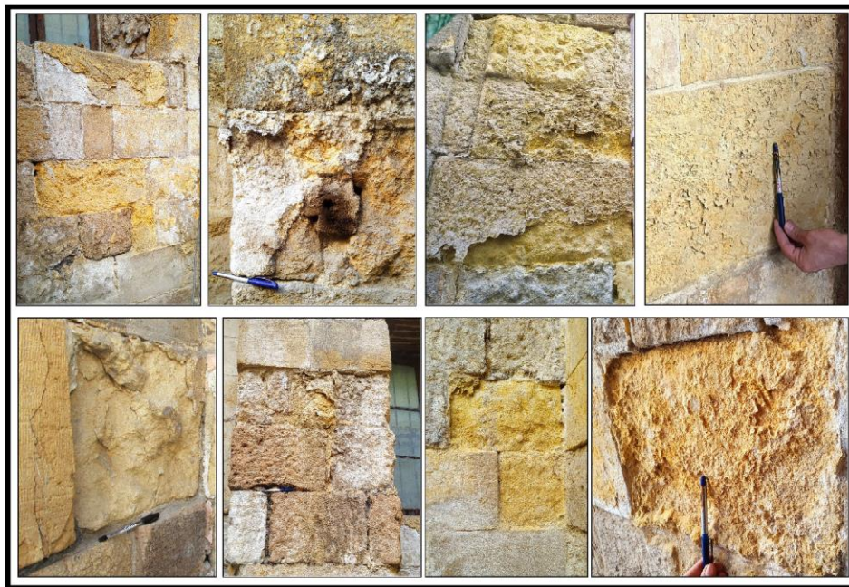
Figure 16: The Spread of the Phenomenon of Flaking and Fragmentation in the Stones of Sabil Muhammad Ali
