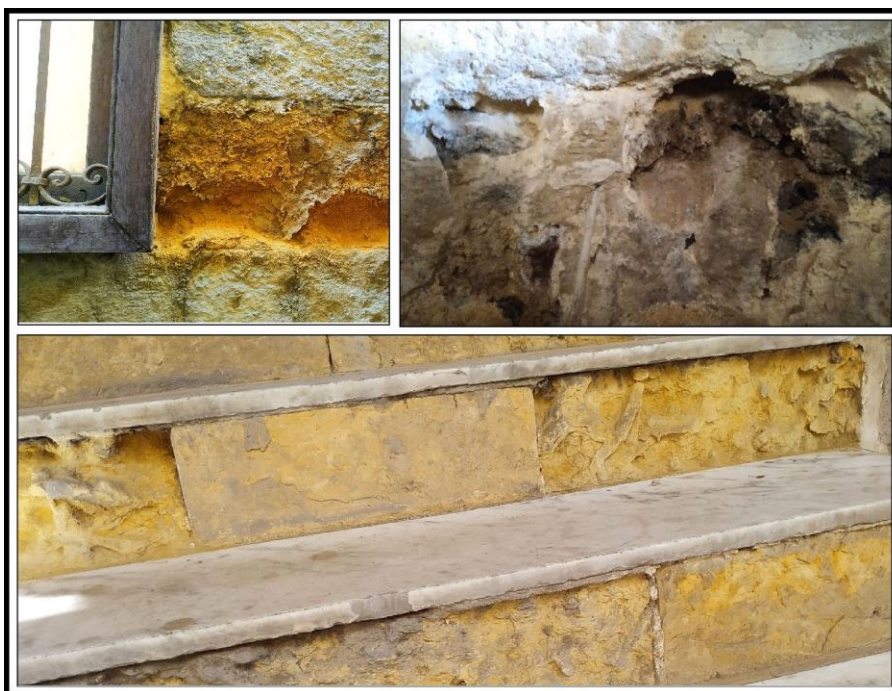
Figure 17: The Spread of Potholes and Gaps in the Stones of Sabil Muhammad Ali
