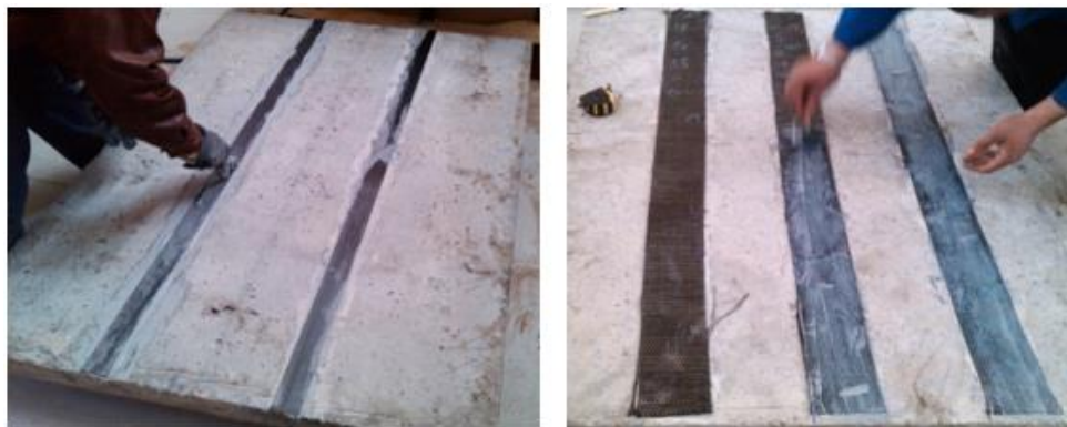
Fig.3 Fixing laminates and Sheets on the Tension Face of Slab.
