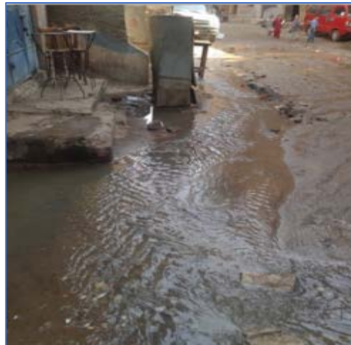
Fig. (7). Deteriorating forms of infrastructure in Izbat Khairallah
