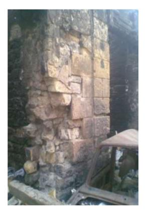
Figure (1) Construction system of the double faced masonry walls in Islamic monuments in Cairo.
