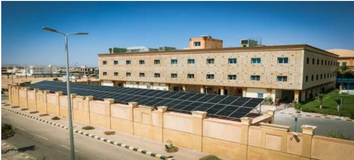
Figure2. Solar Power Stations in Shefaa Al-Orman Hospitals
