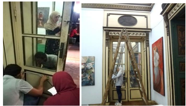
Figure 63. The stage of raising the dimensions of wooden doors. [15]
