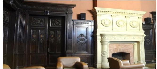
Figure 25. The built-in fireplace is made of artificial stone and signage bricks (refractory bricks). [15]
