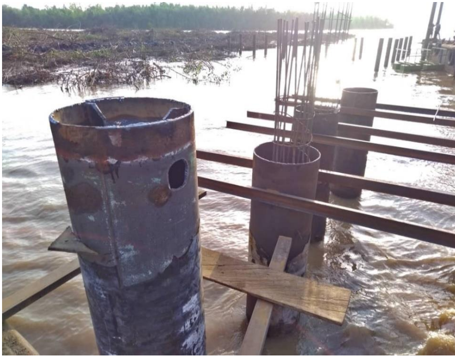
Figure 2: Piles at project site
