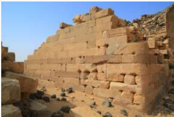
Fig:14 Water outlet building in the main channel.
