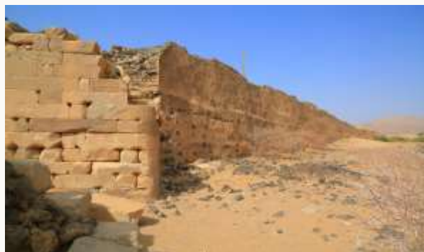
Fig: 10 duct outlet wall (A)
