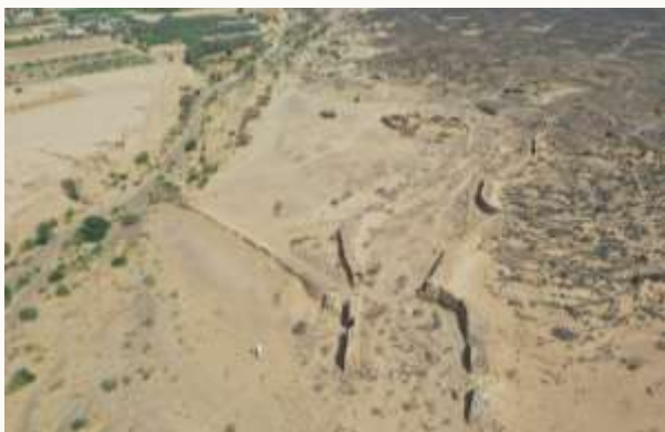
Fig: 7 An aerial view of Wadi Gufaina Dam
