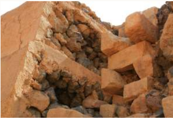
Fig: 13 Building materials in the dam wall from the inside.
