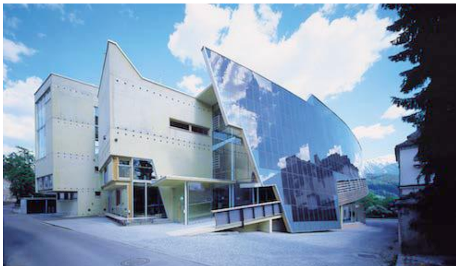
FIG 3: Inclined PV integrated glazed façade of Vocational College in Tirol, Austria Credit: http://www.m9-architekten.at/
