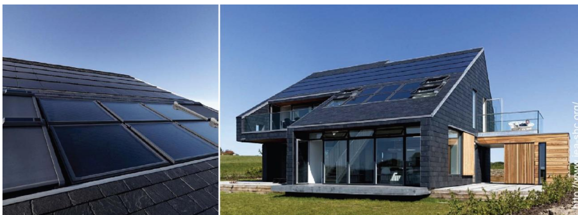
FIG 5: Integration of STC on the pitched roof of single-family house Credit: http://www.iea-shc.org/
