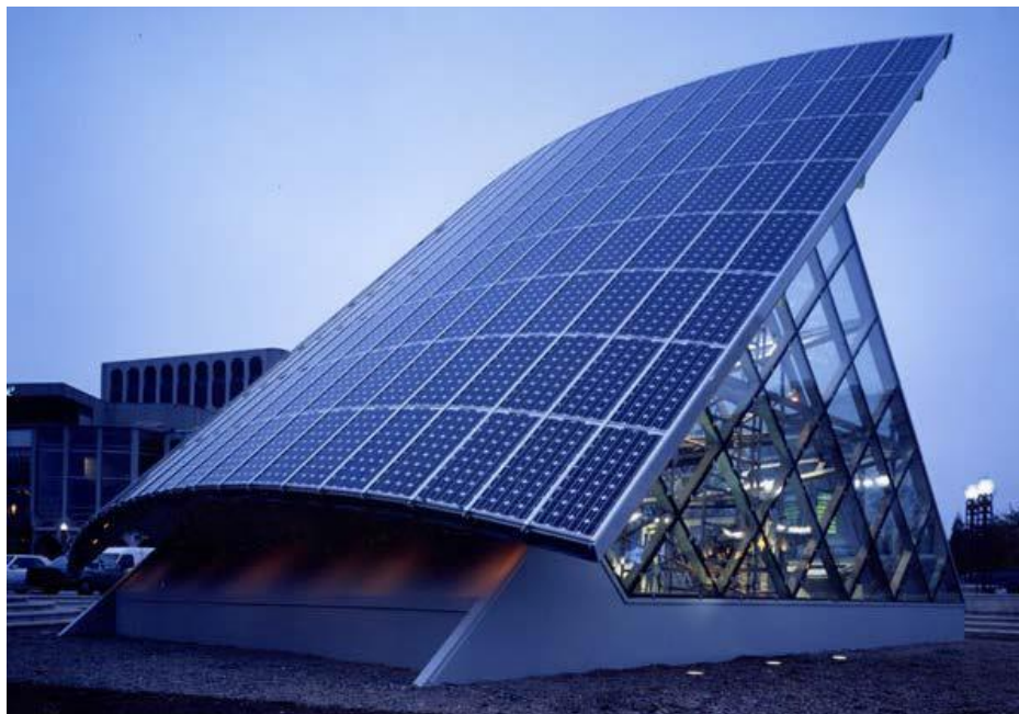
FIG 2: PV integration on the curved roof of BP solar Showcase in Birmingham Credit: http://www.solartechnologies.co.uk/
