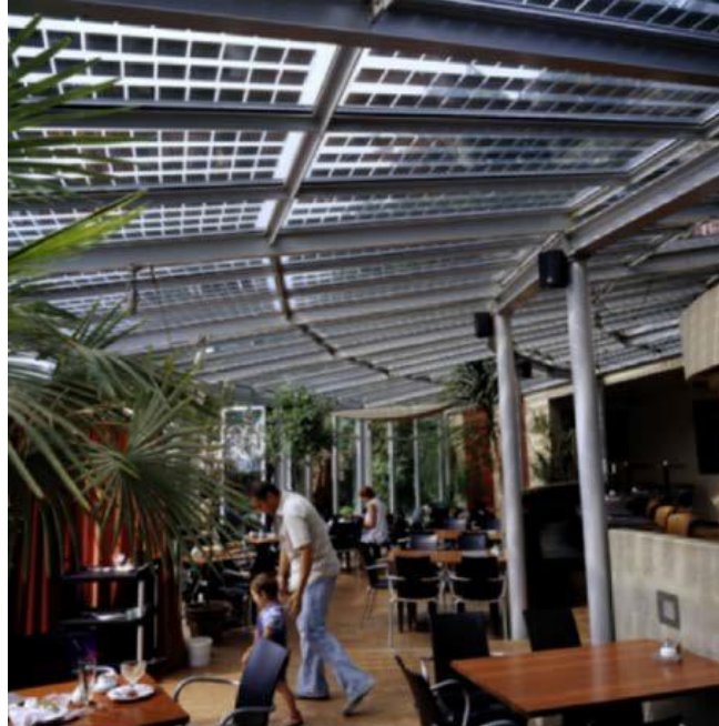
FIG 1: PV integrated double glazed roof of Café Ambiente, Germany credit: http://www.pvdatabase.org/
