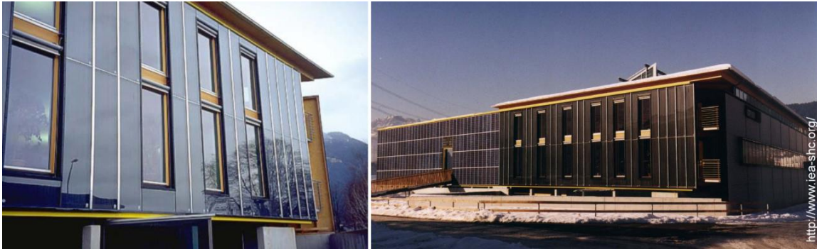
FIG 6: Integrated STC systems on the façade of office building of AKS DOMA Solartedhnik
