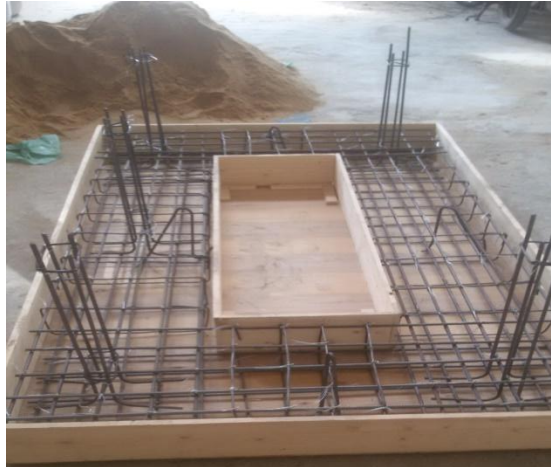
Figure (3): Steel reinforcement of foundation and column indication.
