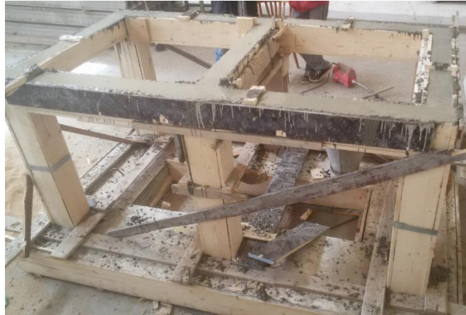
Figure (5): Finishing surface of concrete
