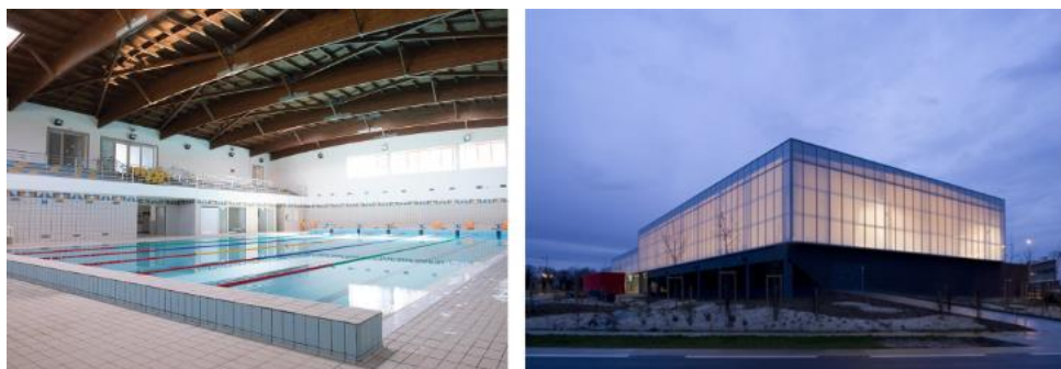
Figure 4 Sports hall, Carquefou, ZAC du Souchais, France (internal and external view)
