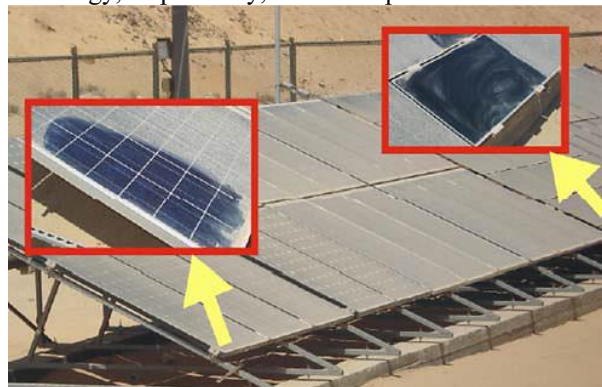
Figure 9: Interconnect cell ribbons, (Left: side shading, Right: bottom shading). [1]
