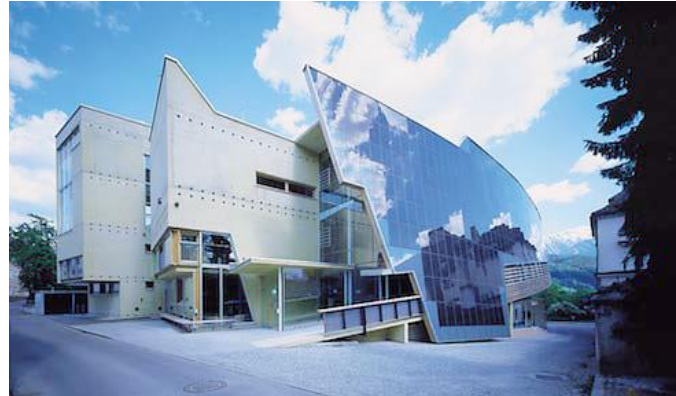
Figure 11: Inclined PV integrated glazed façade of Vocational College in Tirol, Austria [12]
