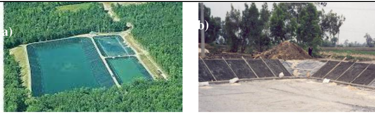
Figure A3: A Stabilization multiple Pond. (b) Single pond at El-Moufty El-Kobra-Kafr El Sheikh Village [19]
