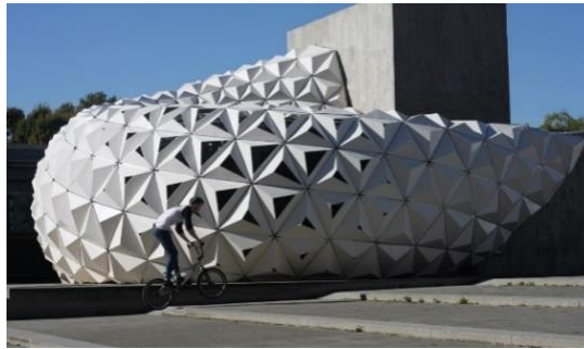
Figure 7 : The ITKE Institute designed and built a new ArboSkin pavilion from 388 bioplastic pyramids. ( Grozdanic. L.,2013)
