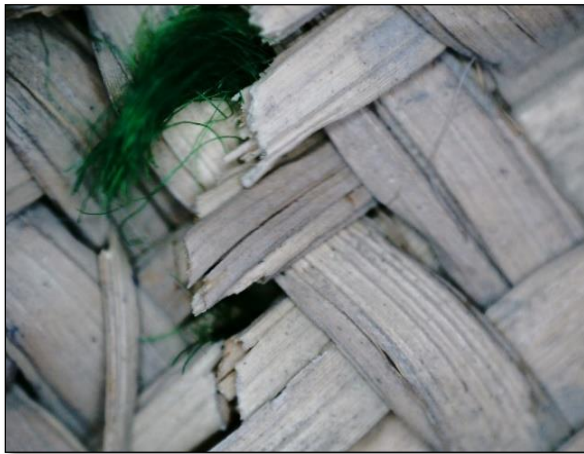
Shape (11) shows corrosion in fiber (zoom strength of 1000X). force of 1000X).
