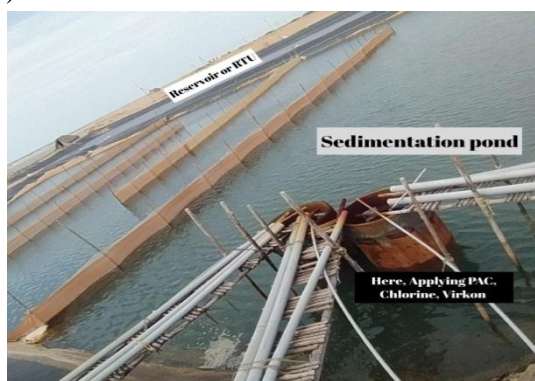
Fig: 3 show the reservoir pond (sedimentation and RTU)
