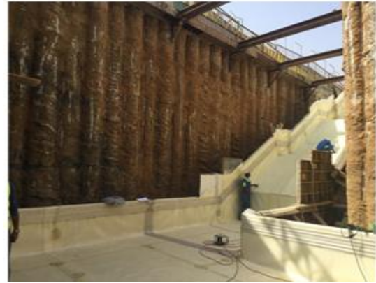
Access (7) contiguous CFA piles
