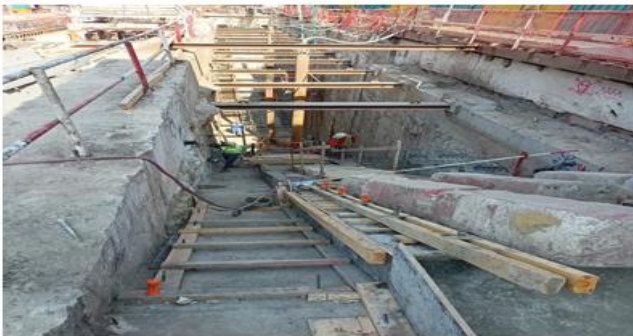
Fig 9. Diaphragm walls in KitKat metro station access
