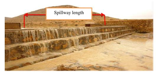
Figure (3): Spillway of the dyke
