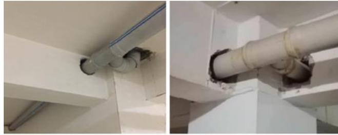
**Fig. 1: Web opening in RC beams.**
