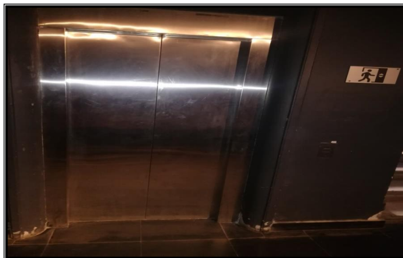
Fig.76. Elevator for Physical Impaired facilities, (researcher picture)
