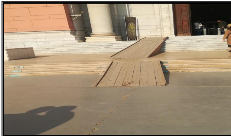
Fig.86. Access Ramp leading to the main entrance of the museum building for Physical Impaired facilities – Egyptian museum in Cairo, (researcher picture)
