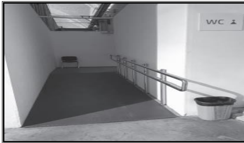
Fig.64. The space is equipped with a low angled ramp and handrails, (Mariya Yasenovska & Olena Zinenko. DEMOCRACY AND HUMAN RIGHTS: BEST PRACTICES OF INCLUSION . PP.1-32).
