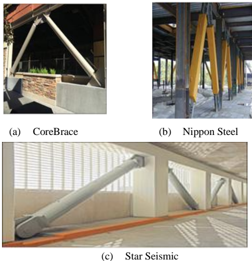
Fig.26. Different BRB shapes
