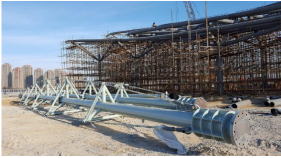
Fig.5. Mega-TTC-BRB Proposed by Guo et al.(2017)[27], [28].
