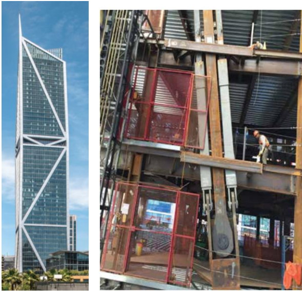
Fig.22. Typical BRBs in Fremont Building [62]
