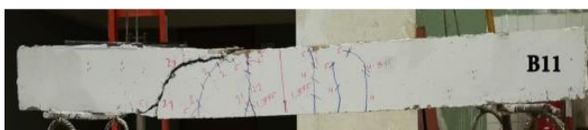
Fig. 10 Pattern of cracks of beam (W1).
