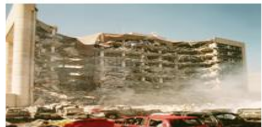
Fig (1.b): Failure of Murrah Federal Structure https://www.bestonlineengineeringdegree.com/the-10-worst-high-rise-building-collapses-in-history/
