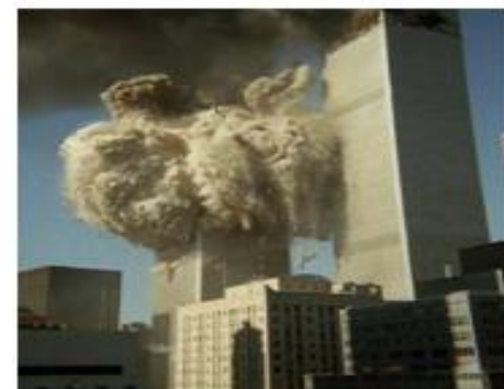
Fig (1.c): World Trade Center Collapse https://www.bestonlineengineeringdegree.com/the-10-worst-high-rise-building-collapses-in-history
