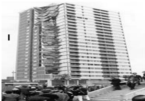
Fig (1.a): Gas Explosions in Ronan Point Building https://community.betfair.com/chit_chat/go/thread/view/94038/29212513/?pg=2&output_method=iframe
