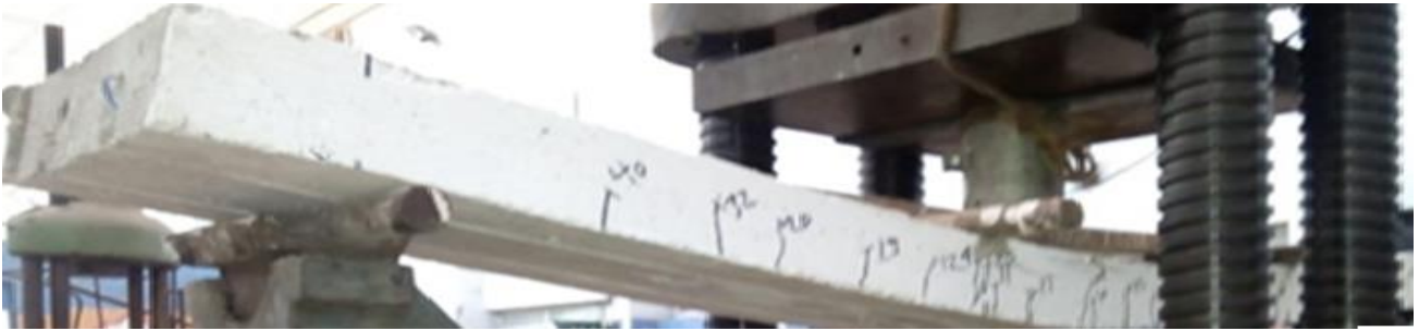
Fig. 9: Crack pattern for RC slab, S-BF-Control
