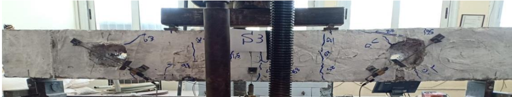
Fig. 5 Brittle shear failure in specimen SO15
