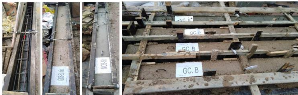
Fig 4.Beam specimens after casting.
