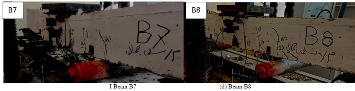
Fig 13. Crack patterns for beams of Group II (reinforced by GFRP bars).
