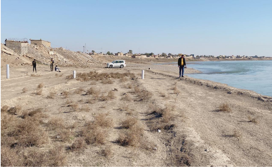
Photo 3: Drilling of wells
