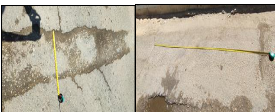
Fig. 14. Utility Patching No.1.
