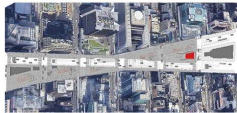
Fig. (8) The development project in 2017 increased the pedestrianization in the street by 50%, allowing more safe space for human activities.
