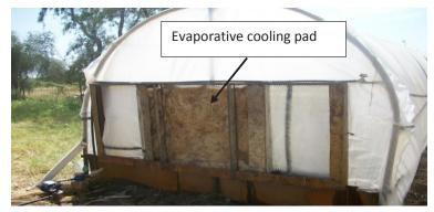
Fig. 2. Position of evaporative cooling pads at one end of the greenhouse
