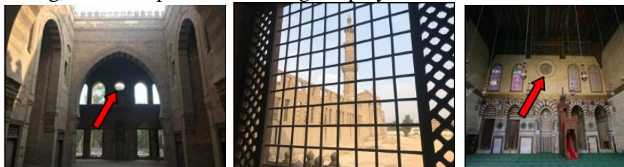
Fig. 6 The position of Qamariya as an urban window in Mamluk religious buildings [author]
