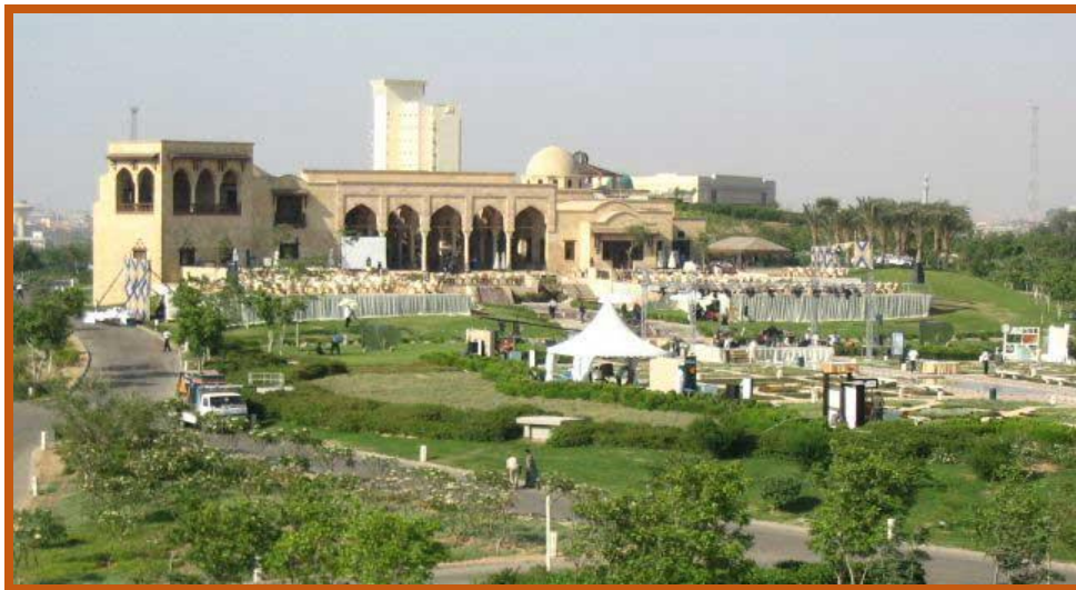
Figure No. (11) shows a general location for Al-Azhar Park, the new green lung of Cairo
