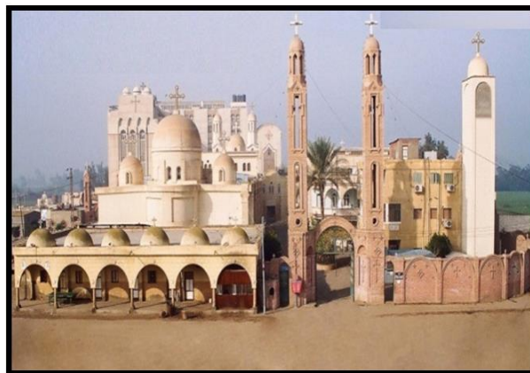
(Pl. 1): An External View of Saint Demiana Monastery at Belqas
