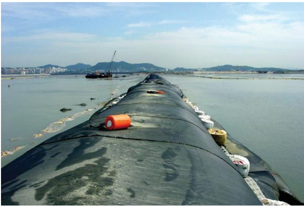
Figure 1: geotextile tube in coastal application, [7]
