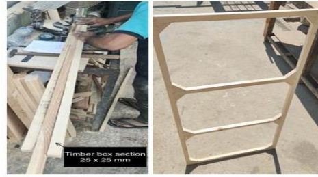
Fig 6. Fabrication of wooden frame
