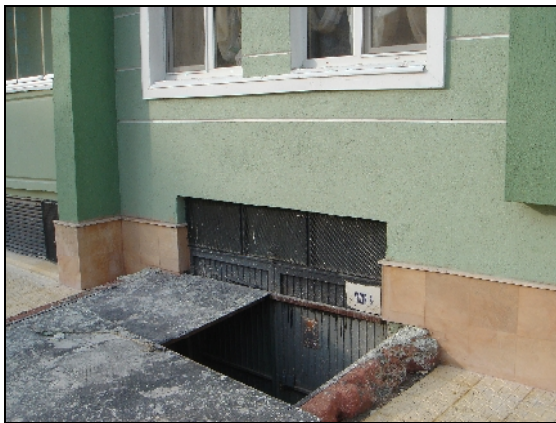
Photo 3. Residential building based on transformer station [Archive of Korur]
